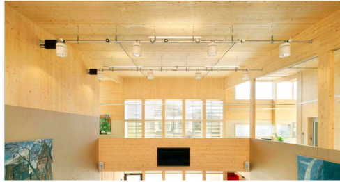
SR example: CLT at Waingels STRUCTURAL
