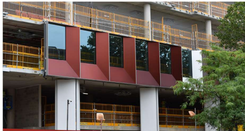
SR example: Prefabricated facade panels, 245 Hammersmith NON-STRUCTURAL
