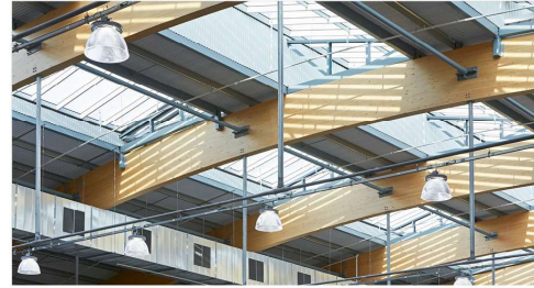
SR example: Glulam beams at Notre Dame School STRUCTURAL
