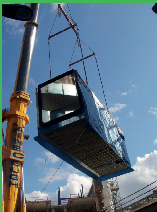
Figure 30 Lifting a room module into place
