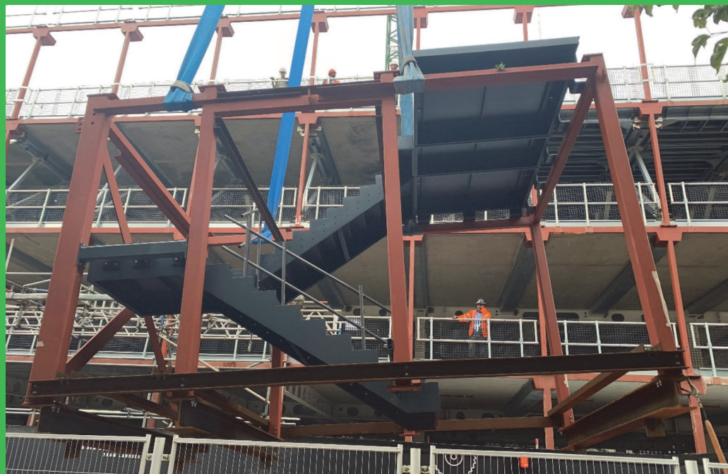
Figure 15 Pre-assembled strongbox core component with integral stairway (courtesy Landsec)
