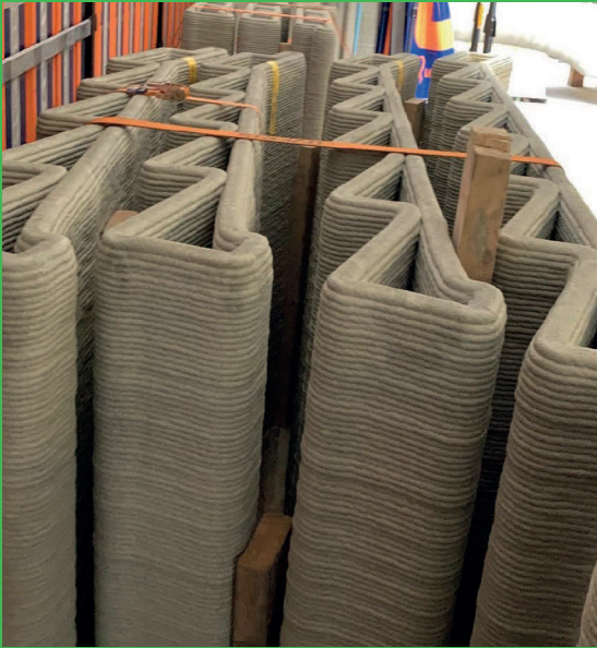
Figure 20 Delivery, installation and completed 3D concrete printed staircase (courtesy Environment Agency)
