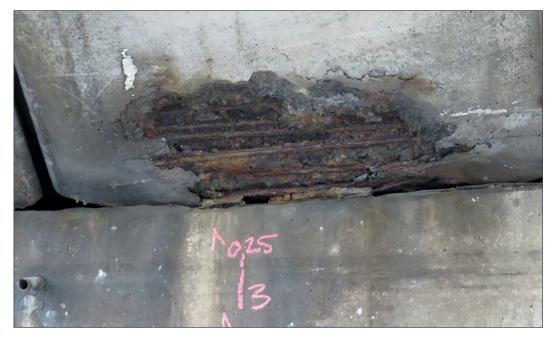
Figure 4 Prestressed beam suffering from corrosion of the reinforcement
