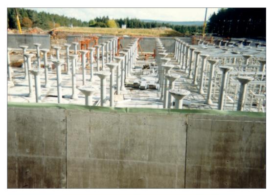
Figure 2 Reservoir constructed using precast wall panels
