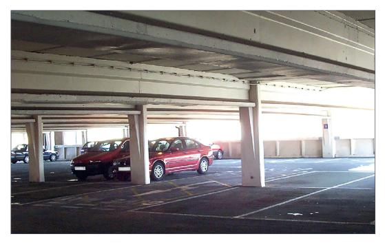
Figure 1 Car park constructed out of precast concrete beams and planks
