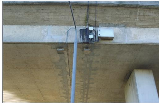
Figure 23 Close-up view of installed ICCP to the underside of a half-joint showing control electronics enclosure and junction boxes
