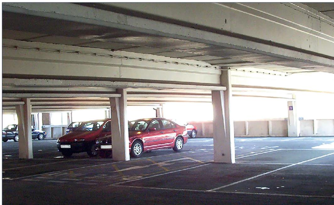
Figure 1 Car park constructed out of precast concrete beams and planks
