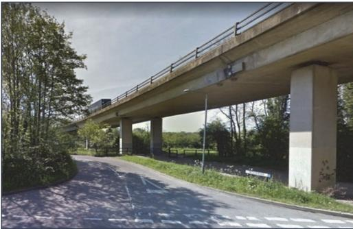
Figure 22 General view of viaduct with ICCP installed to four half-joints
