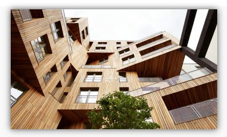
■ The building is a solid CLT structure, manufactured offsite, it uses steel reinforcement where necessary, and is one of the tallest of its kind in Europe
