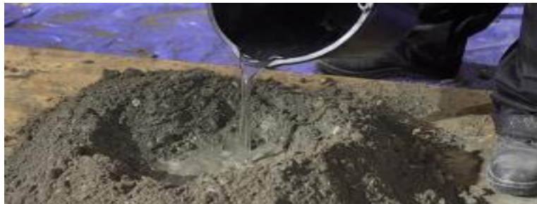
On site mixing for AACM geopolymers materials
