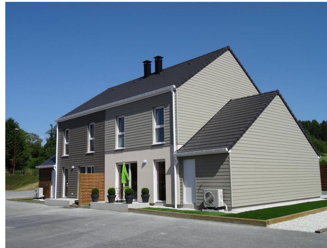
Timber frame for houses
