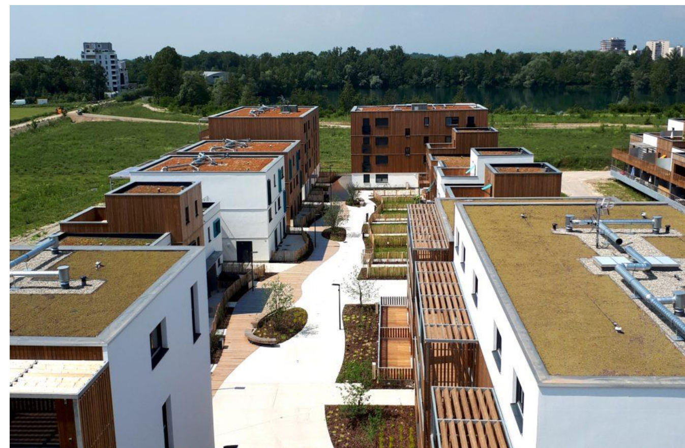
Timber frame for apartments
