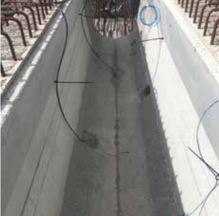
Corrosion protection with AACM on a bridge beam © C-Probe Systems
