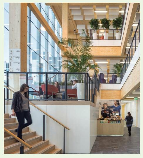
building of this size in Britain, could achieve beyond zero embodied CO<sup>2</sup> emissions. Where concrete is used, it has 100% secondary aggregate and uses the minimum cement through 40% PFA OPC replacement.
