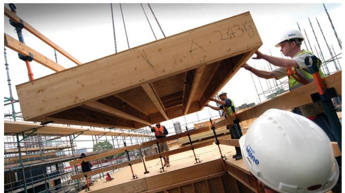
**B) LANDING OF A PREFABRICATED FLOOR CASSETTE**
