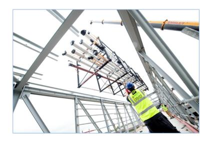
as possible. These modules were bolted together on-site to form a 204 metre run of main services for the new dairy. This equates to close to 70 per cent of the total main services distribution required to operate the dairy.
