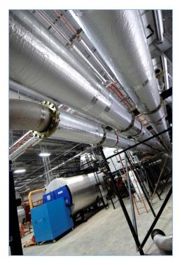
Six heavy duty plant skids, six high level multi-service frames and two heavy duty, floor standing, multiservice frames were also used in the construction of the energy centre. The second phase of NG Bailey's work was installed by a team of two operatives in less than two weeks.
