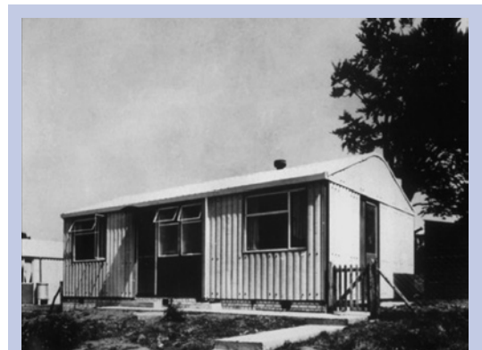
Prefabricated homes after WW2 designed to high performance standards but for a short design life
