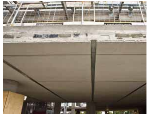
Photos courtesy of Great Portland Estates Example 1 – Precast soffit with reinforced and post tensioned concrete slab above
