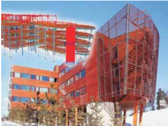
By reducing errors and enhancing information flow, Tekla Structures can make even the most challenging projects, such as Finnforest's Modular Office in Tapiola, Finland, a success story (courtesy of Kingspan Offsite)
