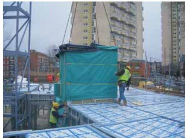
Installation of pod into structural framework
