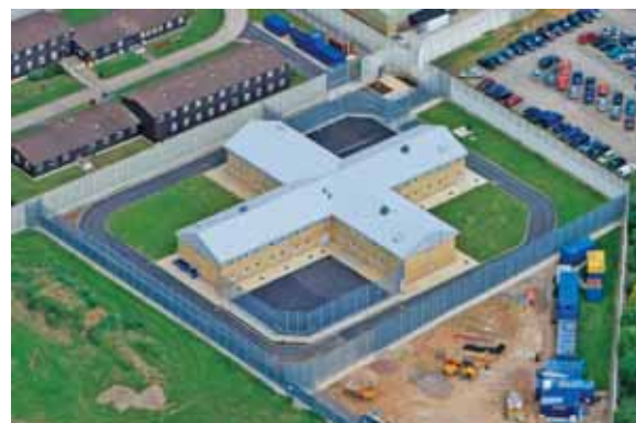
A8 unit at HMP Send
