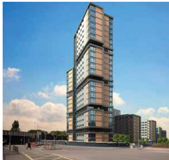
The rapid rise of Europe's tallest modular building
