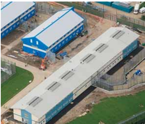
A11 (top left) and double A9 unit at HMP Rochester
