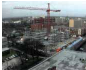
Week 15 - Ground Floor Modules Installation
