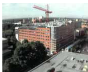
Week 35 - Seventh Floor Installation
