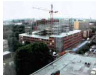
Week 26 - Fourth Floor Installation
