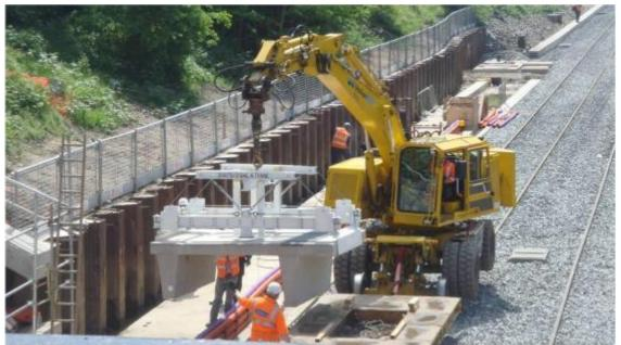
Platform units with integrated surface finish, including warning tactiles, drainage and platform edge coping.
