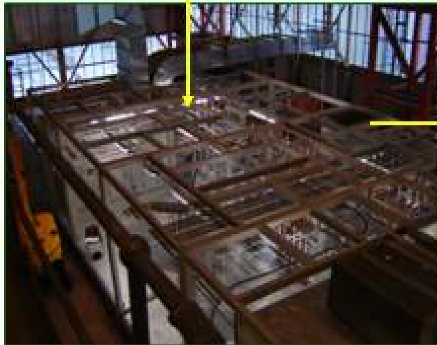
T5a Single Air handling Plant room Modules - strand-jacking
