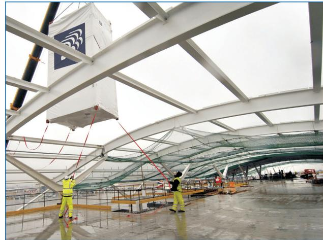
Nodes are structures that connect departure lounges to aircraft, such as the new Airbus A380, to facilitate the quick and easy loading of up to 500 passengers through three separate aircraft doors. Measuring 10m wide by 10m high by 15m long and weighing a total of 90 tonnes once assembled on site, the sheer size and scale of a node presented a unique engineering challenge to the off-site team.
