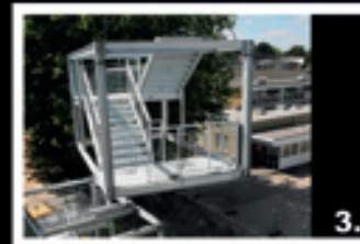
Photo courtesy of Bourne Construction Engineering Ltd
