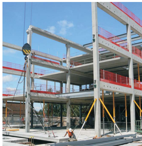
Composite's precast concrete, three-storey structural frame for Phase 2 of a new teaching block at Chessington Community College for the Royal Borough of Kingston-upon-Thames
