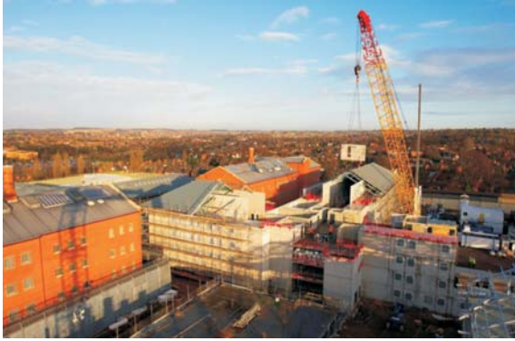
Composite's 346-cell houseblock at HMP Nottingham is of mainly precast concrete, modular construction
